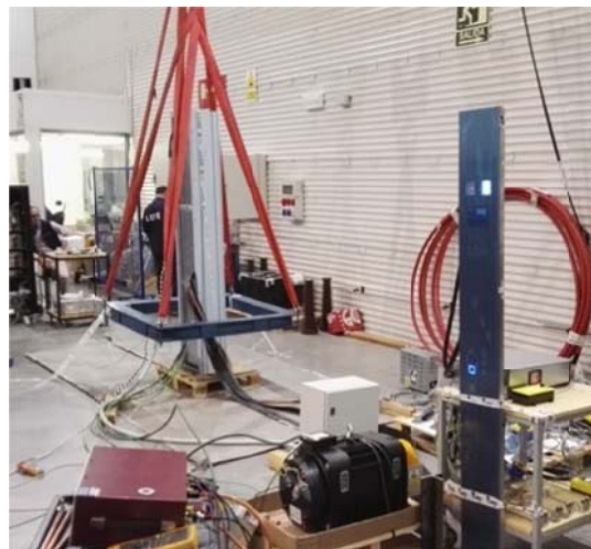
Figure 8: MRL Control panel
